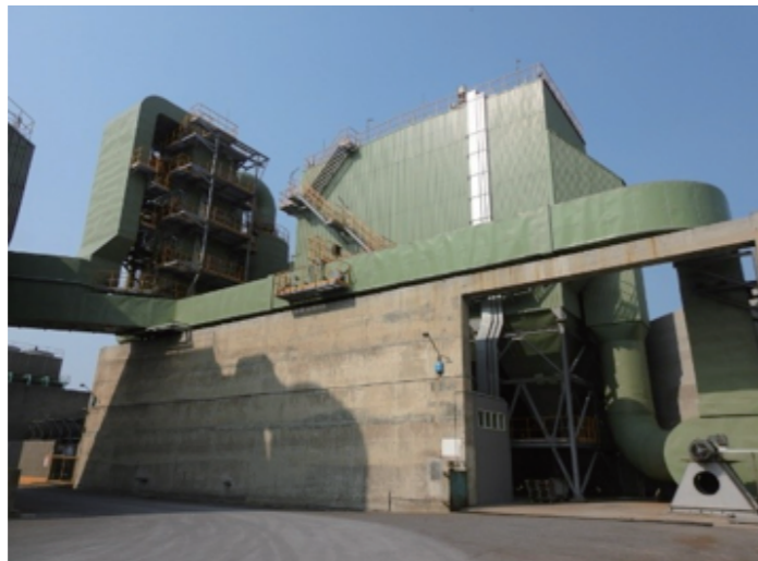
The new Exhaust gas prevention equipment in Lukang Flat Galss Factory
