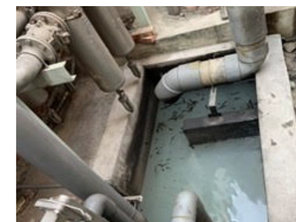
Rainwater and sewage diversion system in Hsinchu Factory
