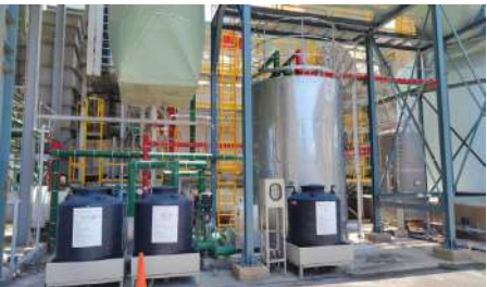
Lukang Flat Glass Factory - Heat-recycling steam boiler system
