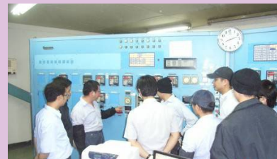
Control room verifies if all is normal
