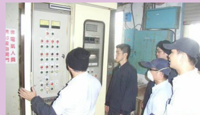
NaOH Spray-Pump & Circulation Pump
