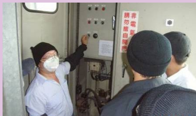
Turn on I.D.Fan
