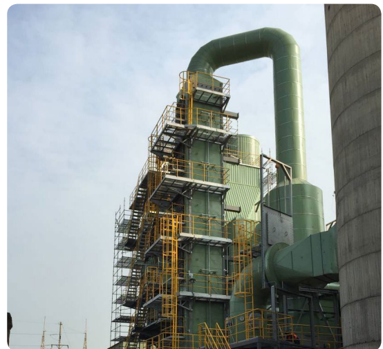
The new exhaust desulphurization system at the Taichung factory
