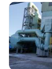
TS-7 SCR denitrification equipment
