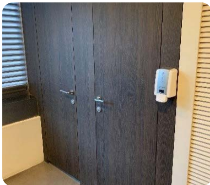
Provide sanitizer in the restroom for toilet seat
