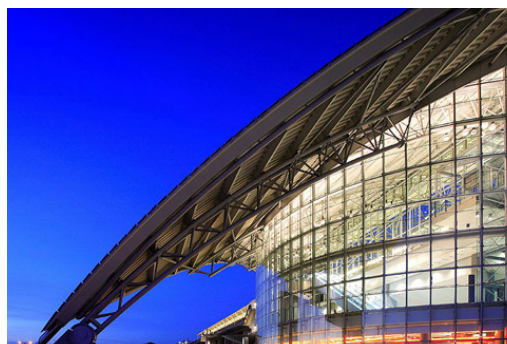
Hsinchu High Speed Rail Station
